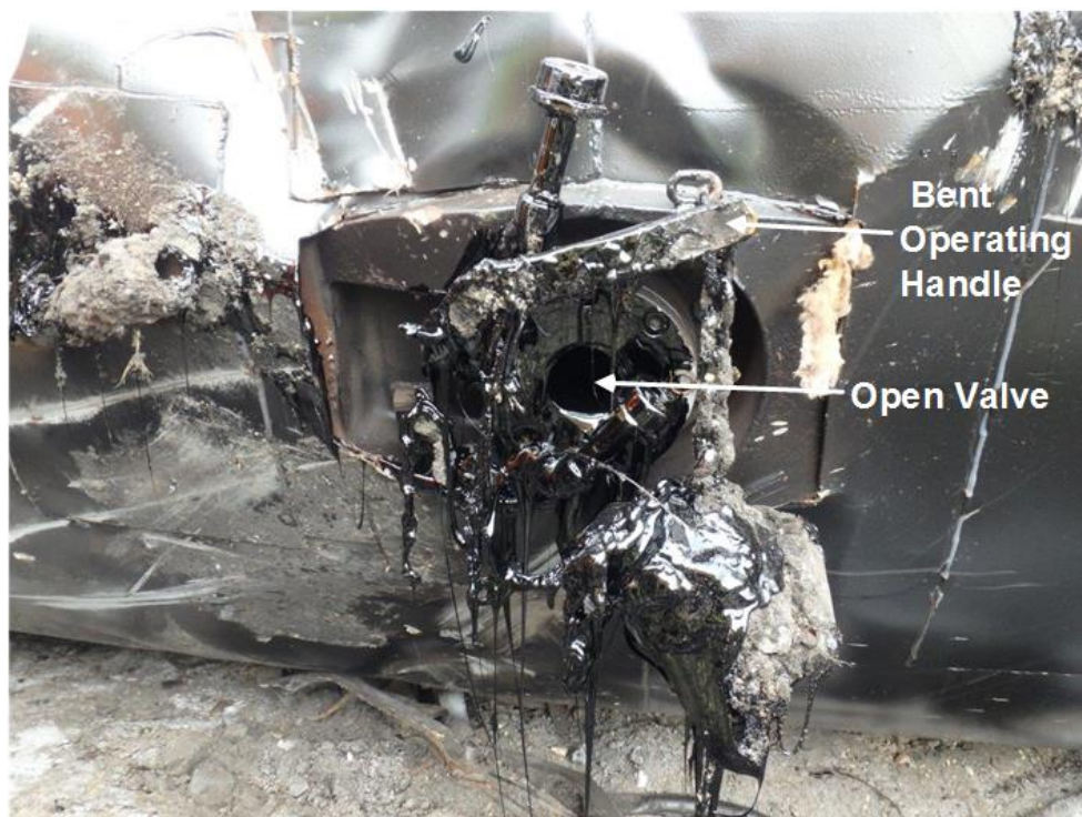
Figure 2: UTLX643949 open bottom outlet valve.
