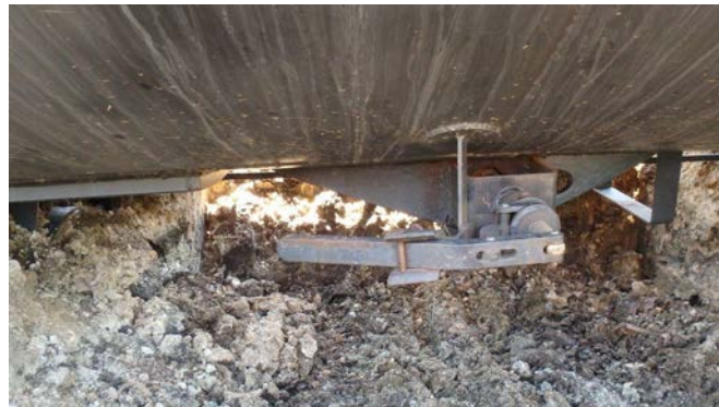
22(d) Undamaged BOV operating handle.
