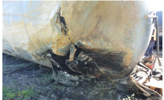
5(b) B-end head dent at 7 o'clock and breach to tank shell where the B-L bolster pad had been attached.
