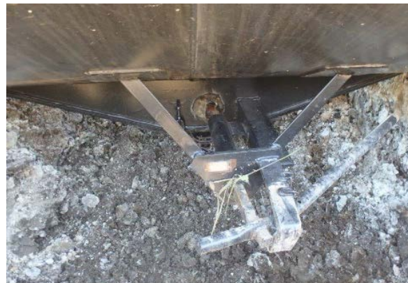
19(d) BOV operating handle was bent, the nozzle was not damaged
