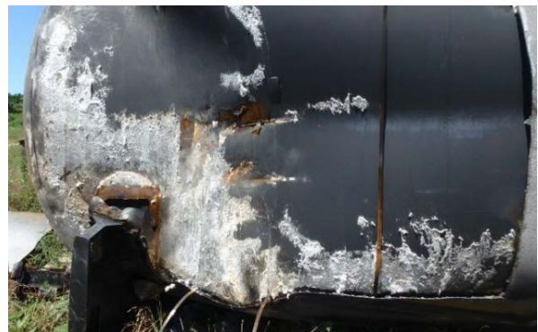
8(d) A-L shell after jacket removal showing non-penetrating gouge and dent left by the impacting stub sill. A-L bolster pad torn from the tank.
