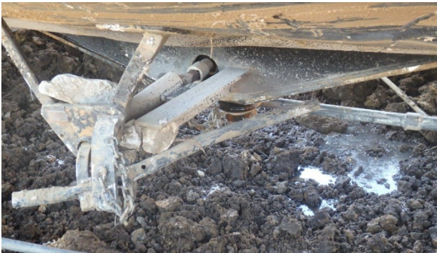
2(c) BOV operating handle and undamaged nozzle.
