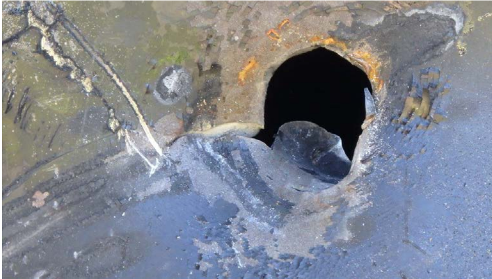
Figure 9. UTLX 209301, 2-inch diameter hole in tank shell.
