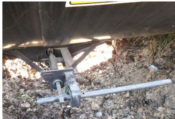
20(d) BOV operating handle and nozzle were not damaged.
