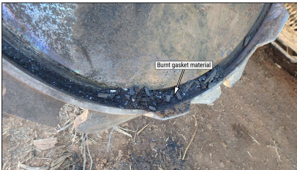
Figure 5. Open manway cover showing burnt gasket material on tank car TILX731739.
