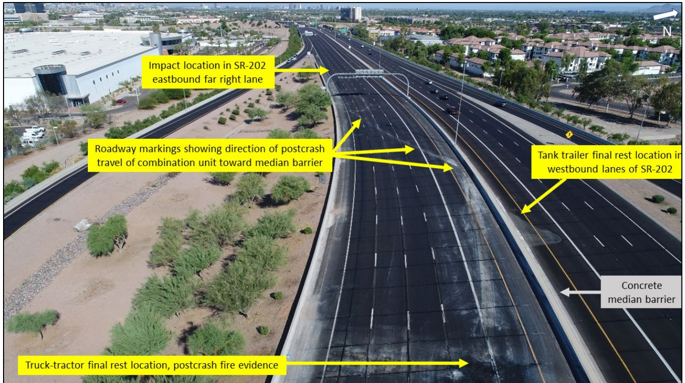
Figure 2. West-facing view of eastbound SR-202 crash location and roadway evidence.
