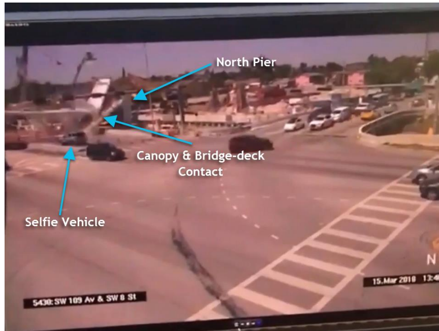
Figure 23. FDOT/Miami Dade camera at frame 39 - 13:46:44.813.
