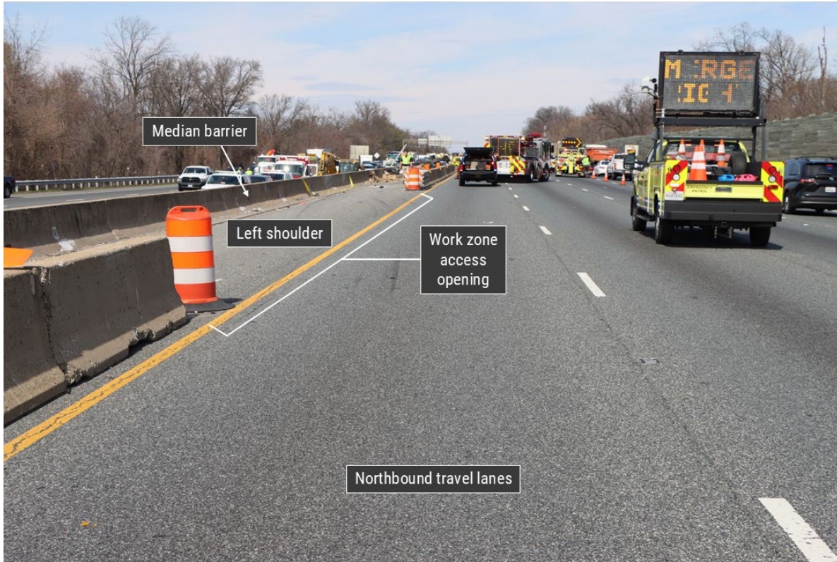
Figure 1. Postcrash view of the work zone and the opening in the concrete barriers through which the Acura entered. (Source: Maryland State Police; annotations by NTSB)
