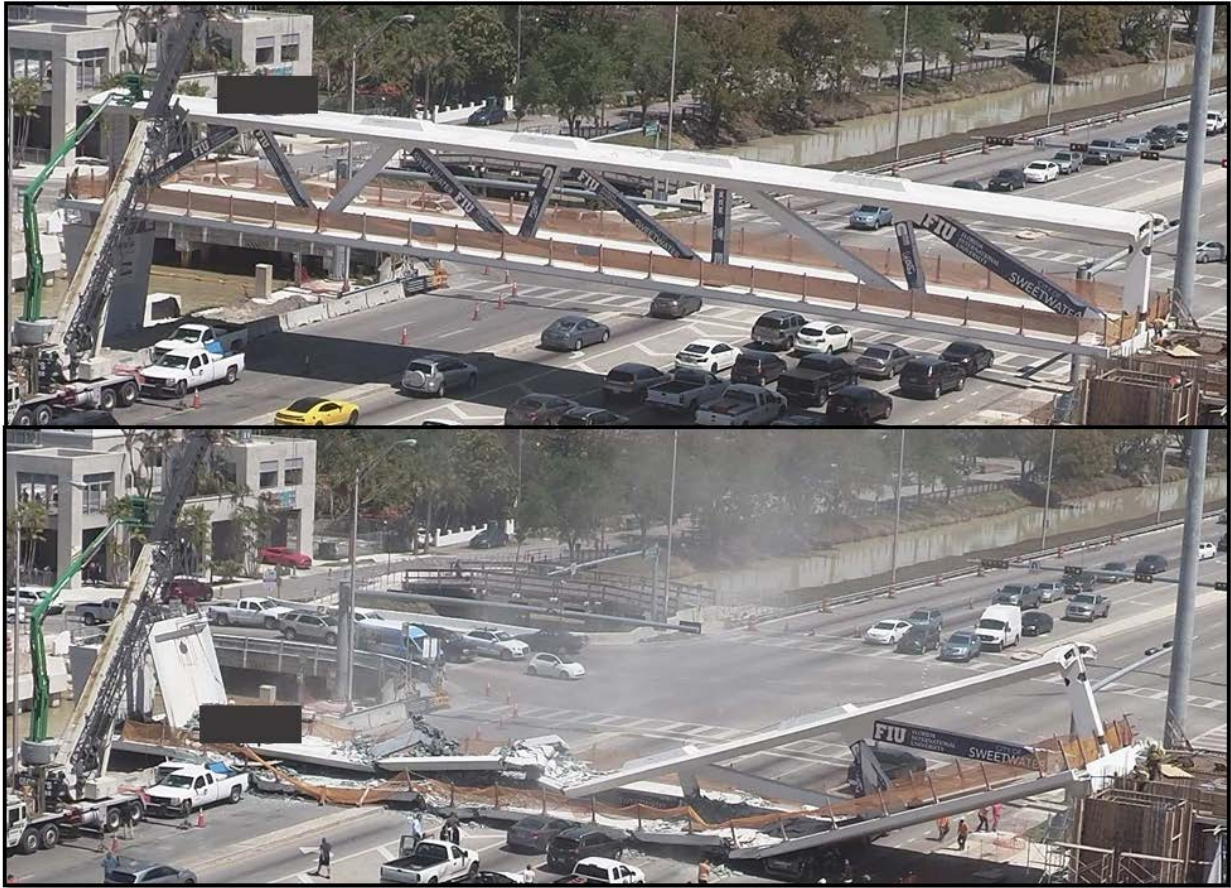
Figure 4. Still images from FIU parking garage camera, showing east views of pedestrian bridge, March 15, 2018, precollapse (top) and postcollapse (bottom). (Source: FIU video camera)
