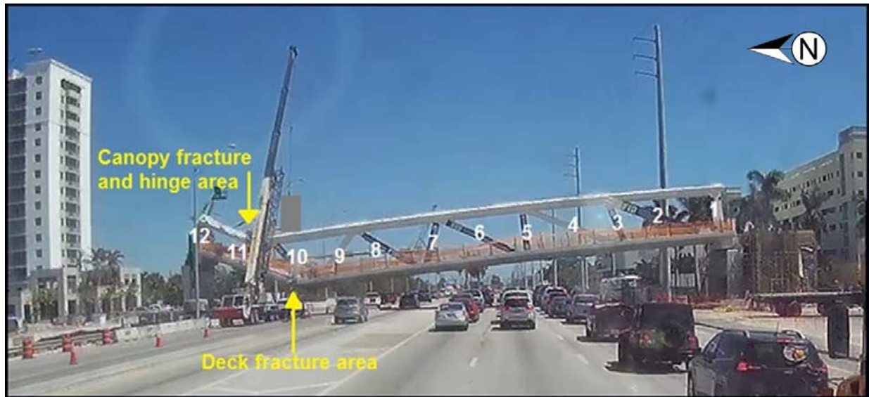
Figure 10. Still image (time stamp 13:46:44:046) from in-vehicle mounted video camera on pickup truck traveling east on SW 8th Street, showing full-width canopy fracture and deck fracture areas at north end (pylon pier), March 15, about 1:46 p.m.
