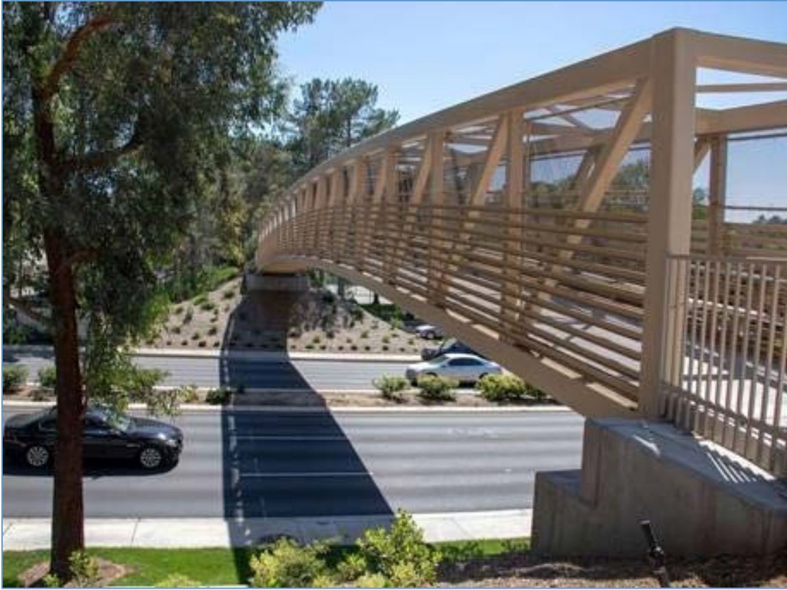
Figure 8. Typical truss bridge with one set of regularly spaced vertical truss pieces running along each side, with top lateral bracing constructed of steel. (Source: Santa Clarita, California )
