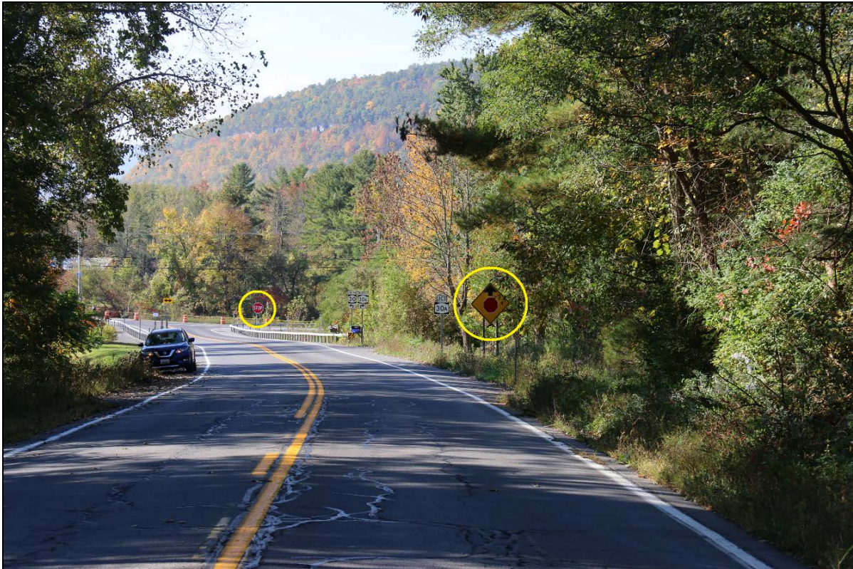
Figure 5. Southbound approach view of NY-30/NY-30A intersection about 660 feet before intersection. (Stop ahead warning sign and intersection stop sign are circled in yellow.)
