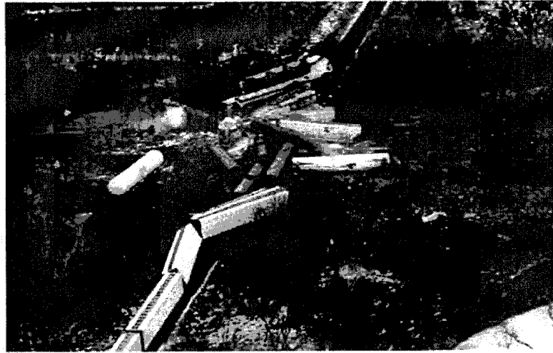
a) Aerial photograph of the Minot ND Derailment [6].
