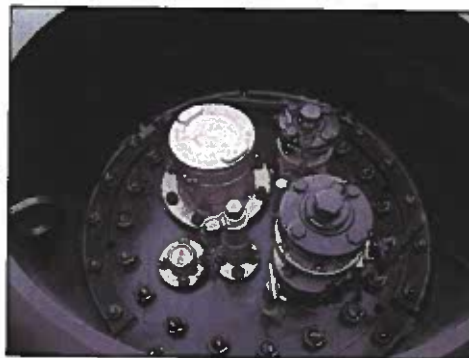
Typical arrangement found in the protective housing on the CPC-1232 and DOT-117 cars.
