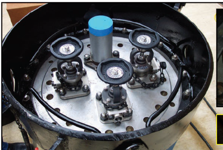
New valve arrangement for Chlorine and other service
