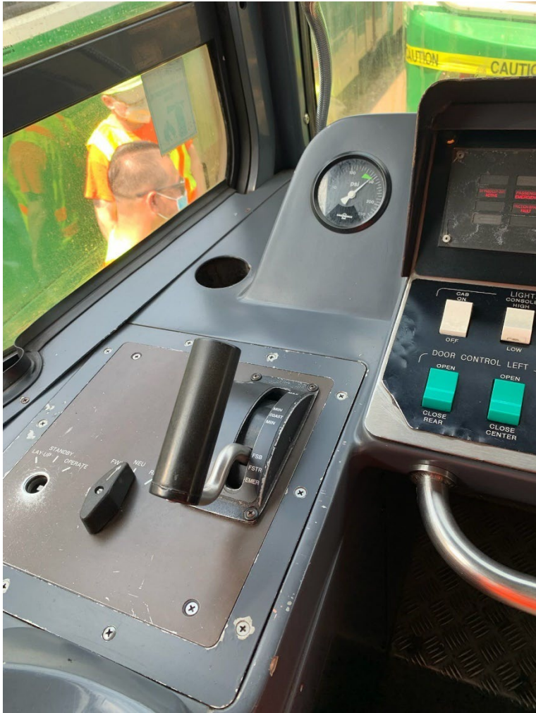
Figure 4: Photo of master controller inactive, “deadman” switch not engaged. Source: NTSB
