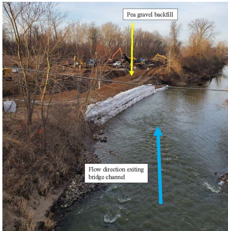
Figure 1 - View Looking Southwest from Edwardsville Road Bridge (Photo Taken 17 March 2022)
