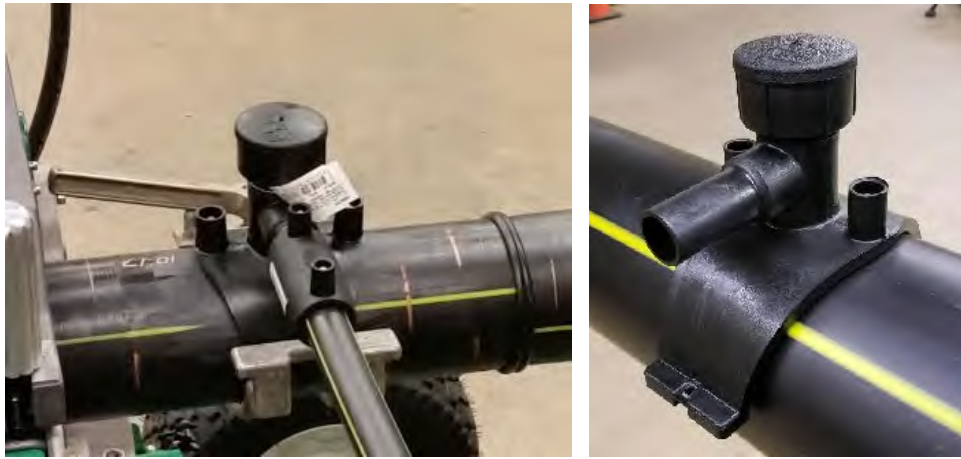
Figure 35.20.30-1 Service Connections to PE Mains
