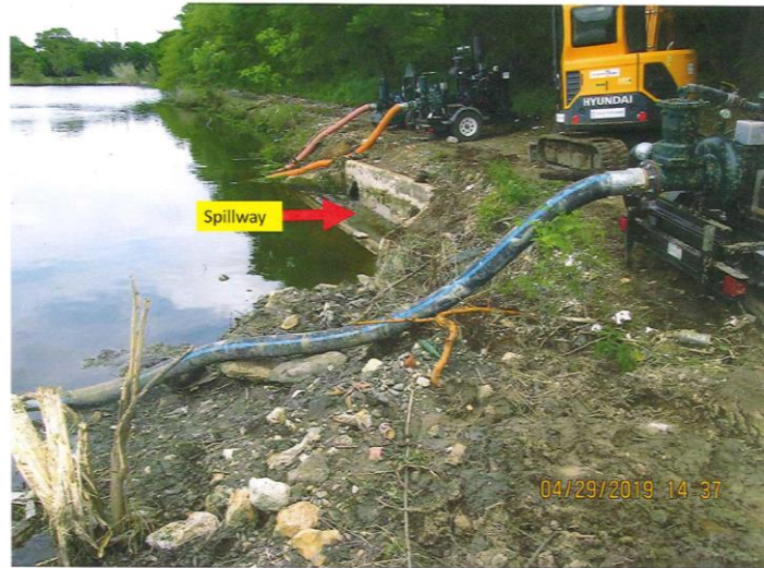
Figure 2: Echo Lake spillway, post-accident drainage pumps are present in the photograph.
