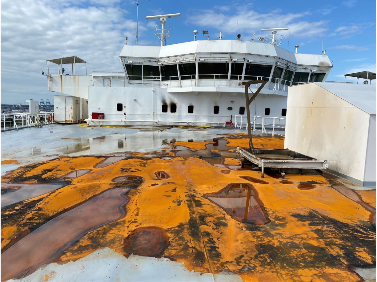
Figure 42. Thermal damage to the deck at the bow.
