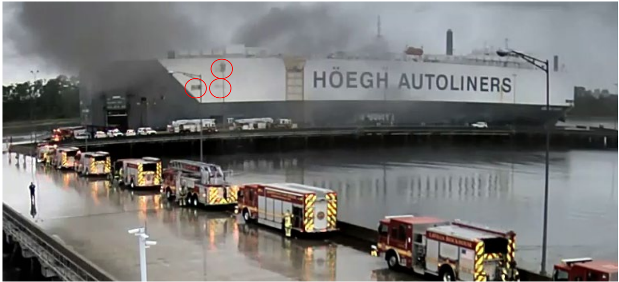
Figure 34. Thermal discoloration (circled in red) of the paint approximately 14 minutes after E48's arrival.
