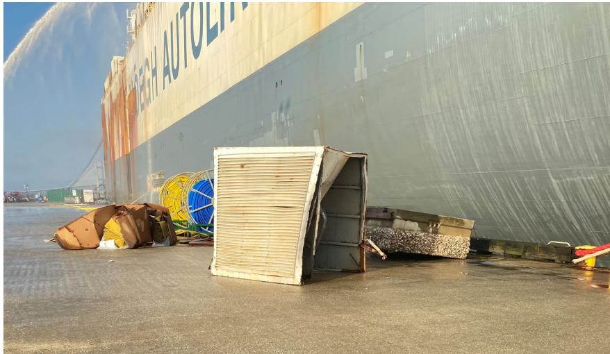
Figure 22. Ventilation doghouse from vent 10E on the starboard side of the bow found on dock.
