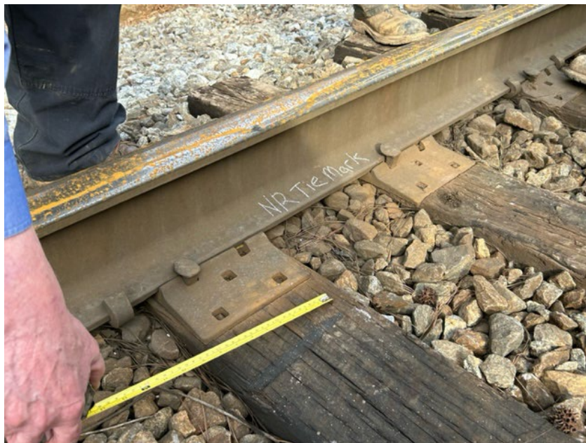
Figure 3. View of wheel flange marks on cross-ties near the north rail.
