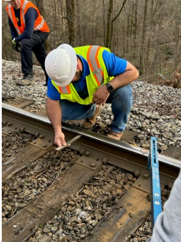
Figure 5. Investigator measuring alignment (degree of curvature).
