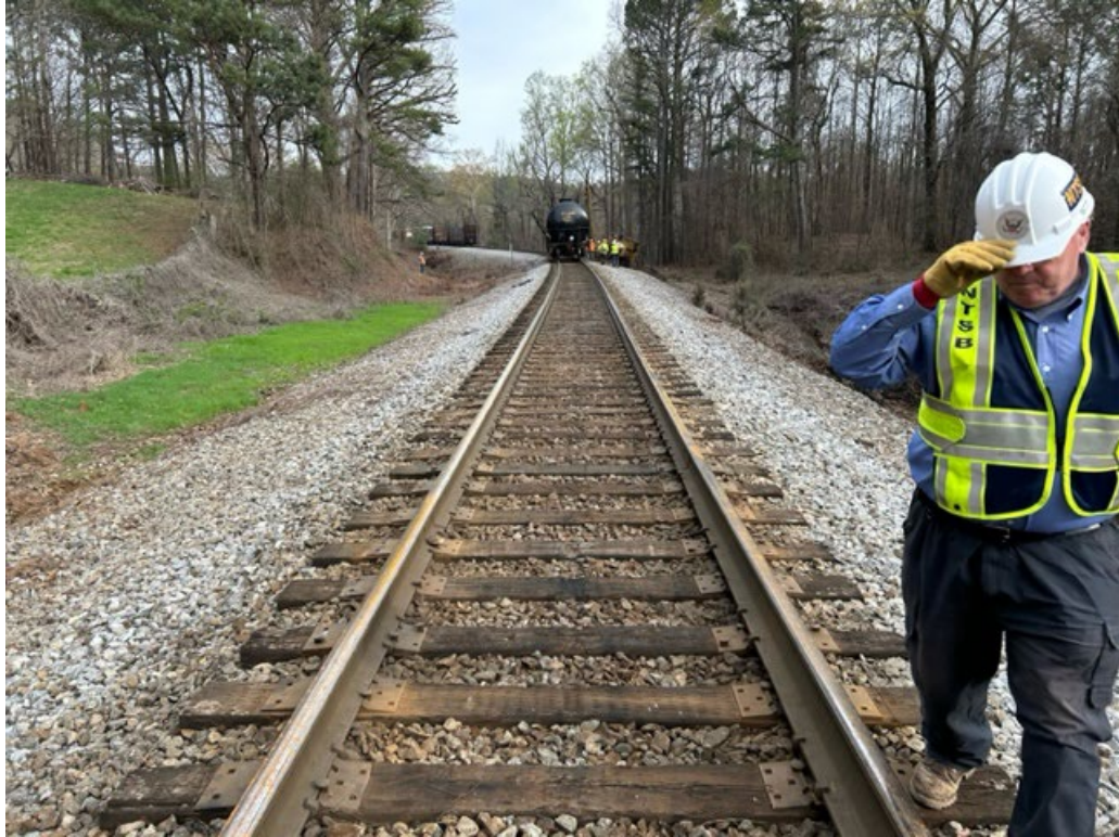
Figure 7. General view of the track looking eastward.
