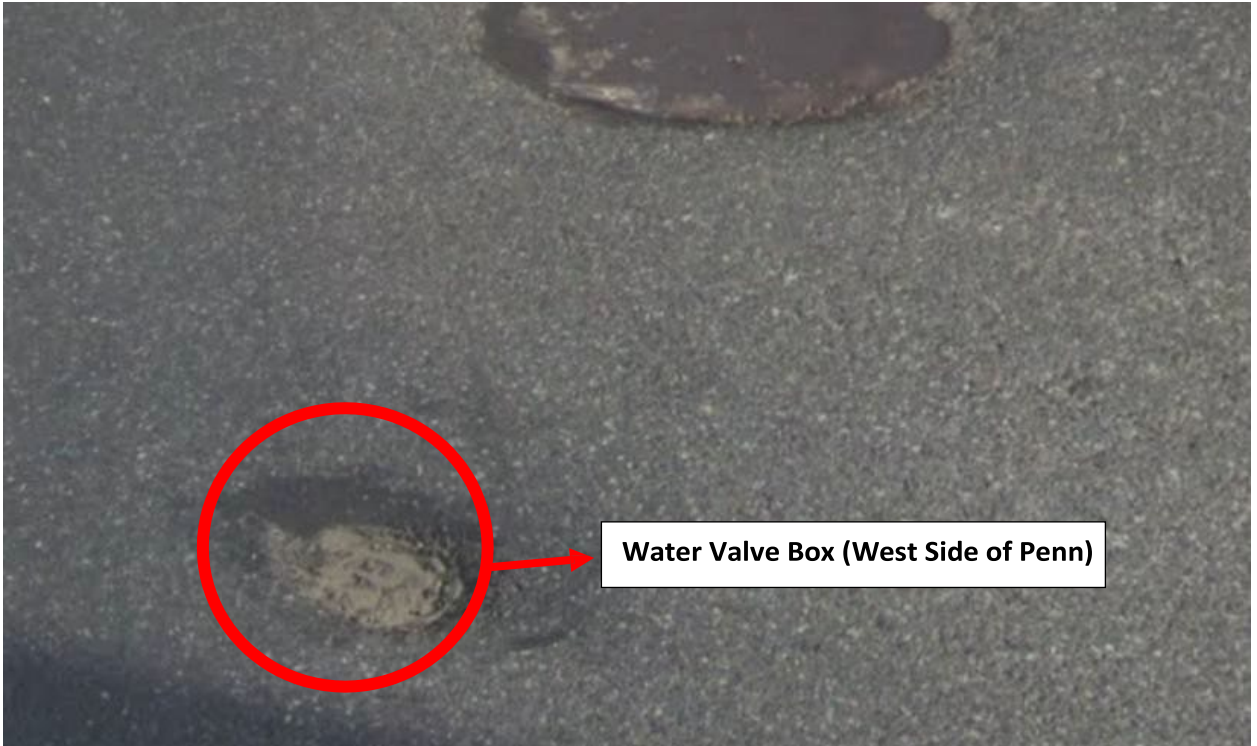
Figure 3: Close up of a water valve lid from a 2018 google photo (Photo courtesy of UGI)
