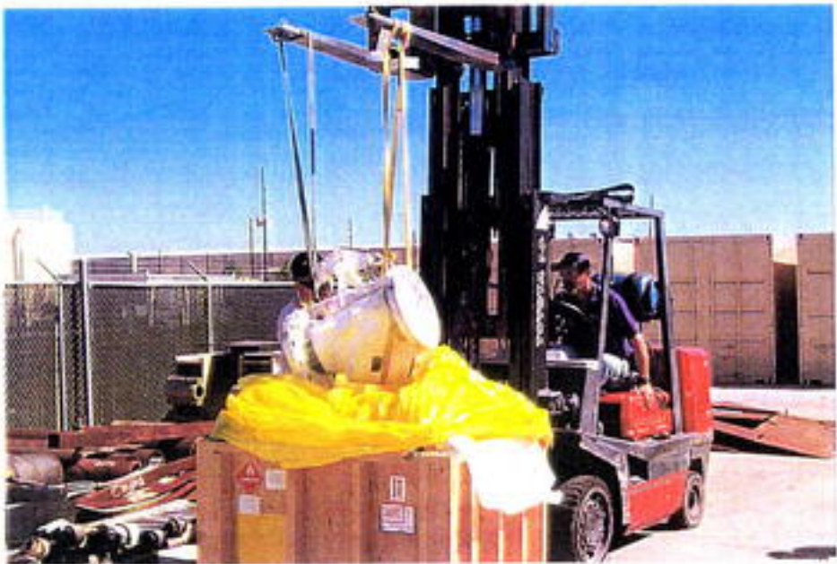
Figure 2.6 Removal of Valve From Crate
