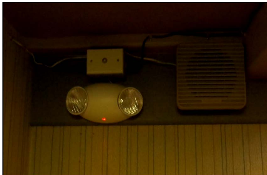
18 19 Figure 3. Bunkroom emergency lighting on board the similar vessel Vision . The lighting was of the 20 same make and in a similar location as was on board the Conception . Also note the public address 21 system speaker to the right of the lights.
