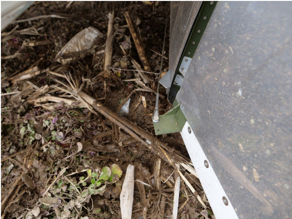
Figure 9 - Lower right side of rudder, cable attachment point
