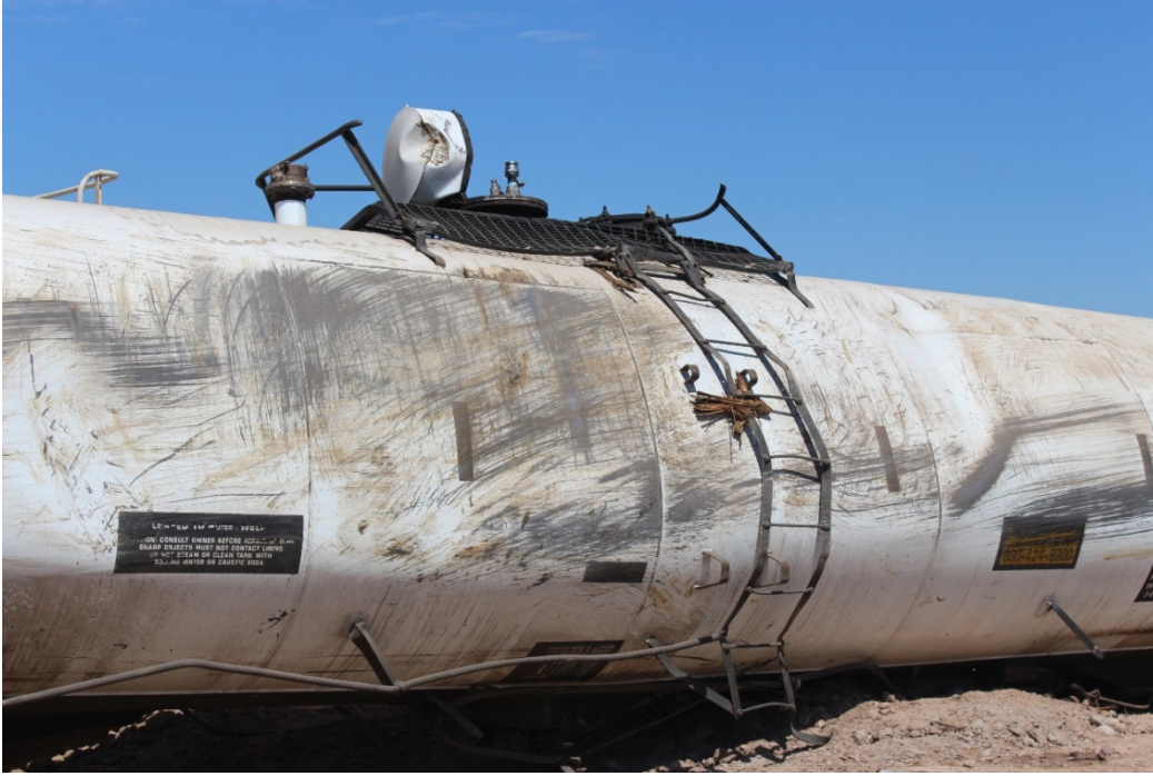
Figure 5: ACFX 72540: Dents on left side and PRD housing (photograph courtesy of PHMSA)
