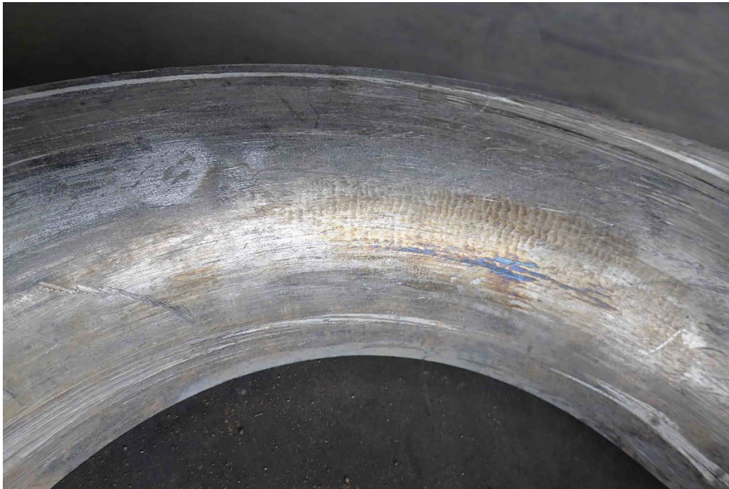
Photo 59 - Number 2 compressor shroud inner surface
