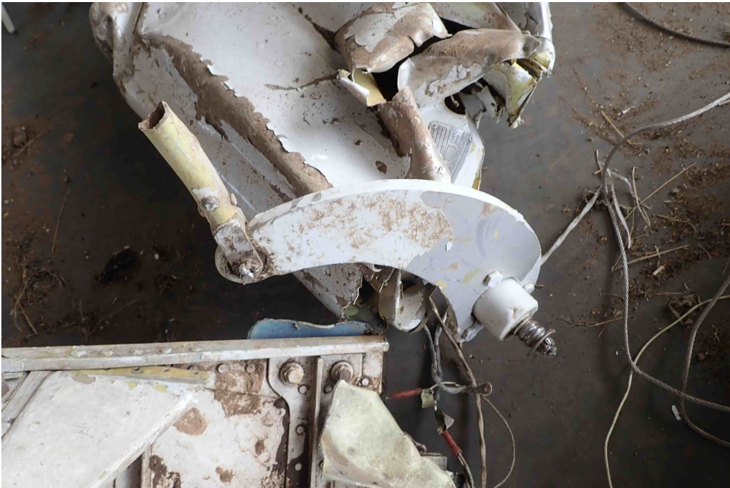
Photo 39 – Elevator control horn
