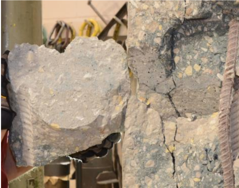
Figure 4.15. Construction joint interface of Specimen 1 (as-placed, cracked) after failure.
