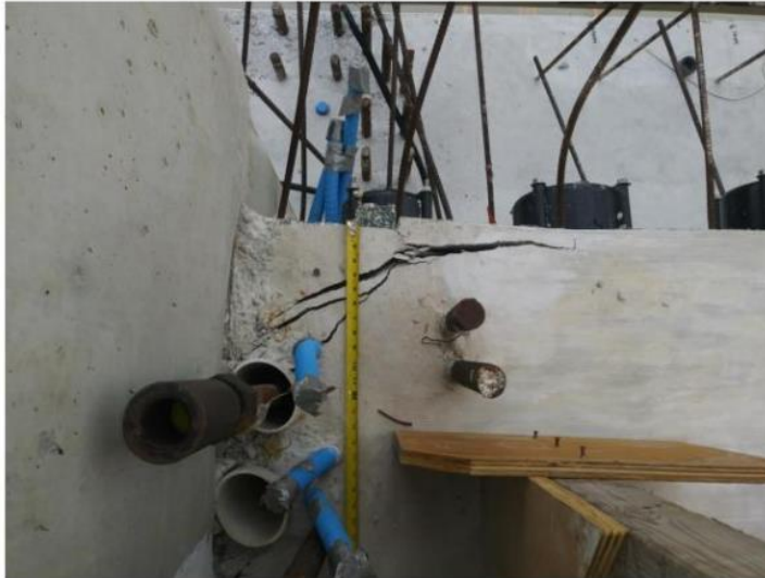
East side of Member 12. Photo taken March 12, 2018 by MCM.
