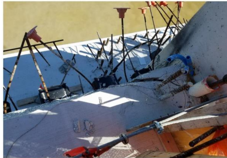
West side of Member 12. Photo taken March 13, 2018 by BPA.
