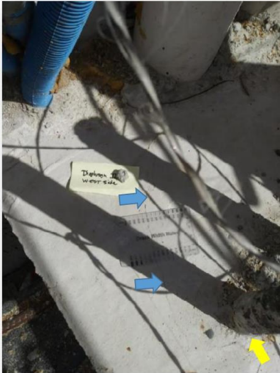
Photo 12 from BPA crack inspection after formwork/scaffolding removal. February 28. Crack is indicated by blue arrows. Crack width ruler appears to indicate 0.014 inches.
