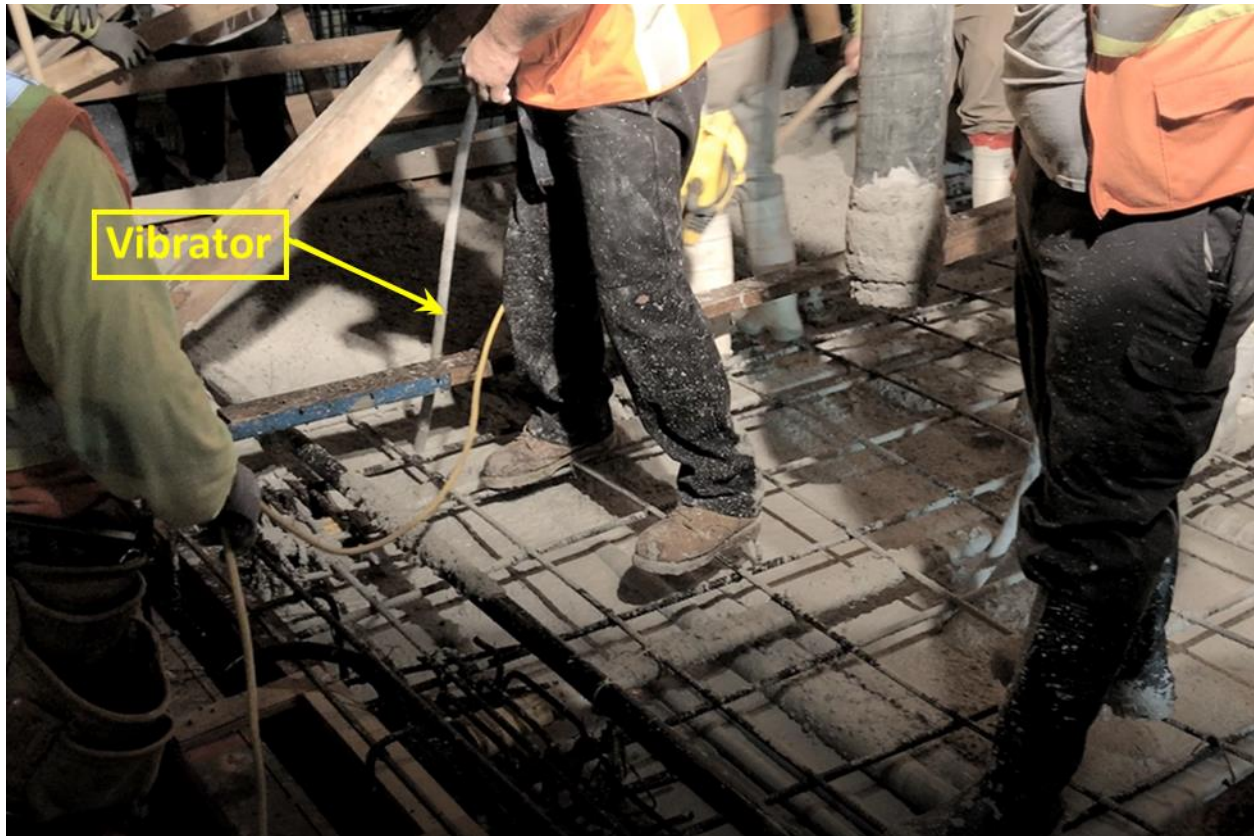
Figure 3.4. Screenshot of video of first deck concrete placement attempt.
