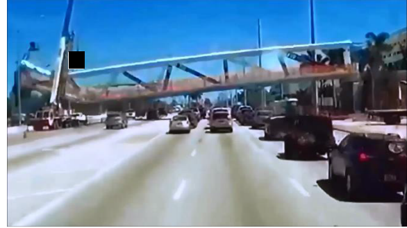
Figure 2.4 Video frame during collapse
