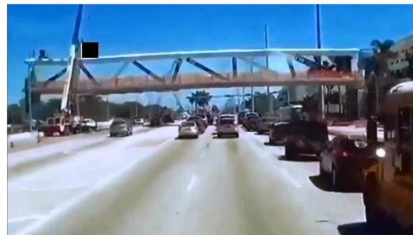
Figure 2.2. Video frame during collapse
