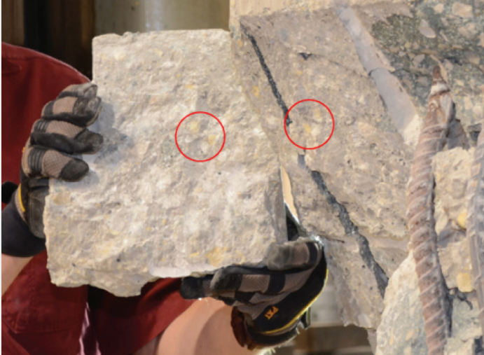
FIGURE 6-30 Construction joint interface surface after failure for a roughened specimen. Circled areas show corresponding fractured aggregate on each side of the joint interface. (Source: WJE)
