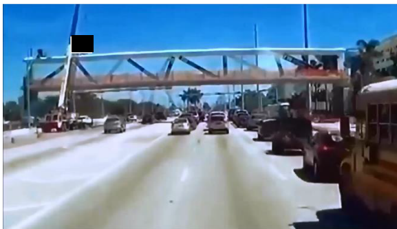
Figure 2.1. Video frame at start of collapse
