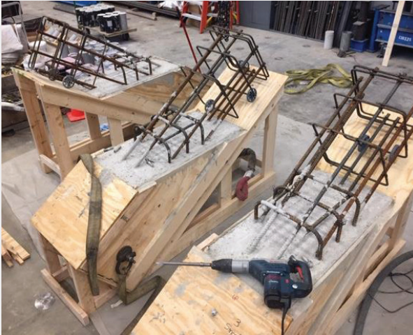
FIGURE 6-21 Lower half of test specimens cast at same angle as member 11 connection to the bridge deck. The lower half is analogous to the bridge deck. Note the electric chipping hammer used to roughen the surface of the roughened joint specimens. (Source: WJE)
