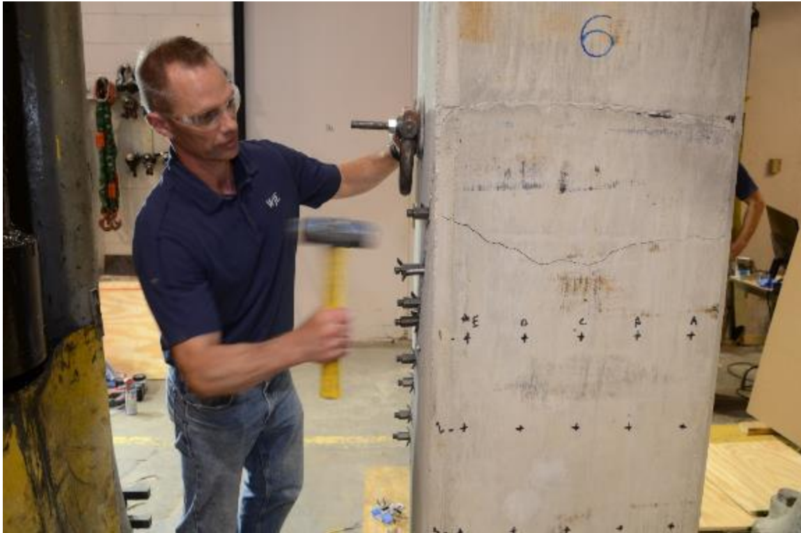
Figure 4.9. Stone-splitting wedge sets being used to create a crack across the construction joint of Specimen 6
