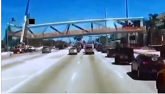
Figure 2.3. Video frame during collapse
