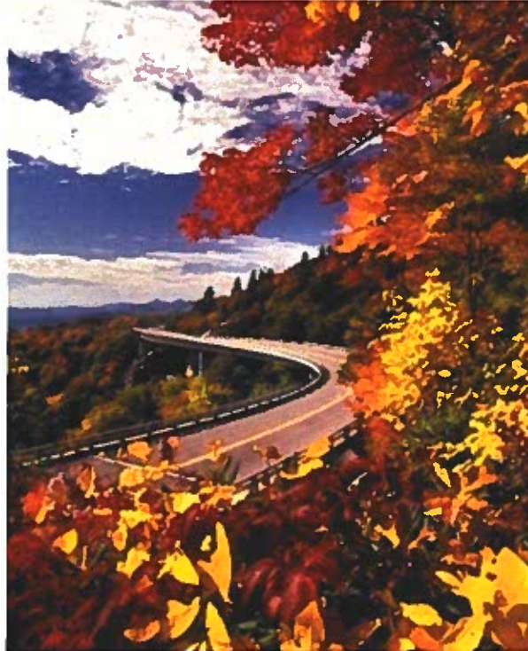
Blue Ridge Parkway Viaduct, NC National Park Service
