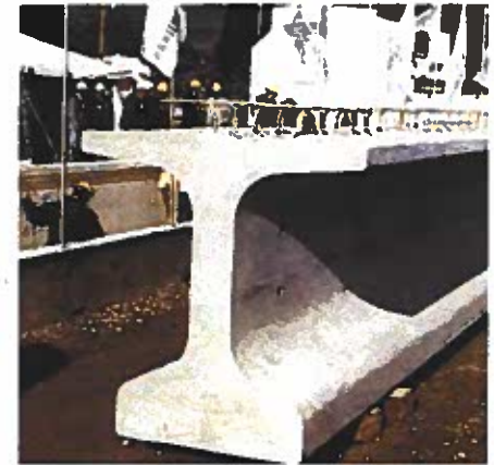
Typical Precast Concrete I-Beam
