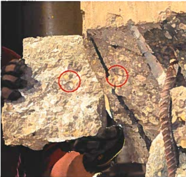
Fractured Aggregate Roughened Joint Interface
