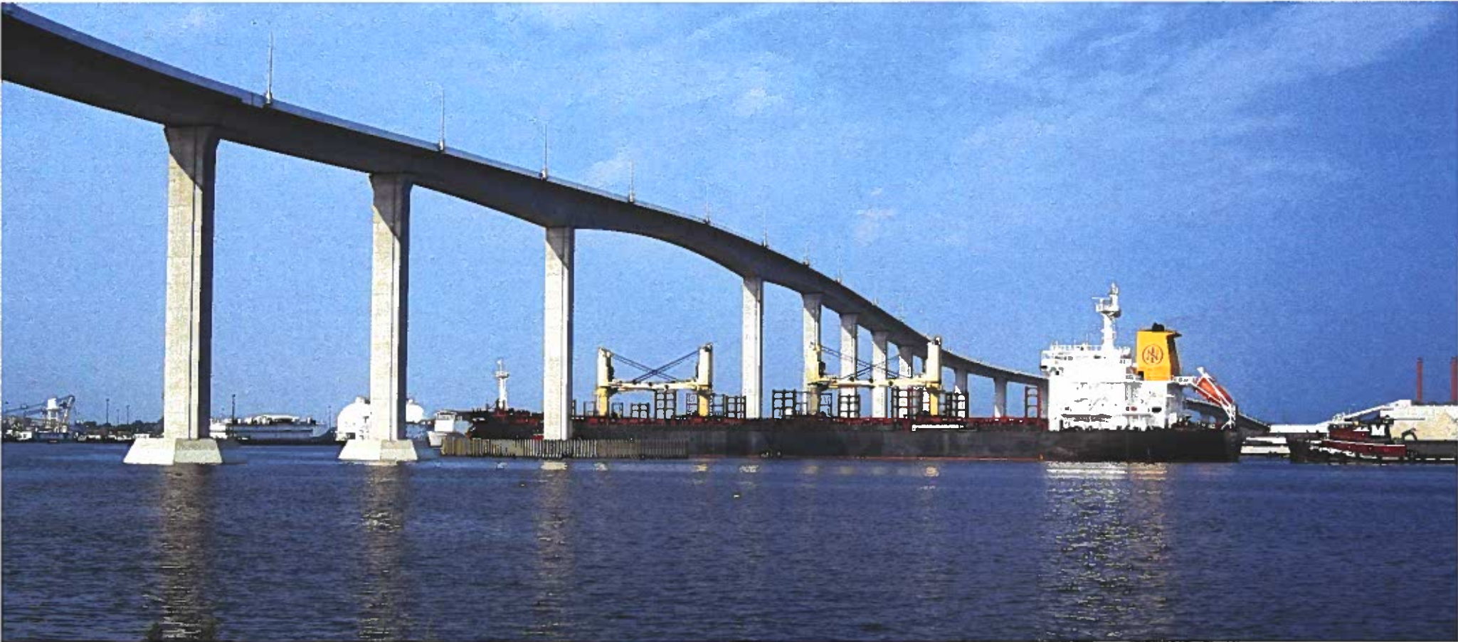
South Norfolk Jordan Bridge, Chesapeake, Virginia
