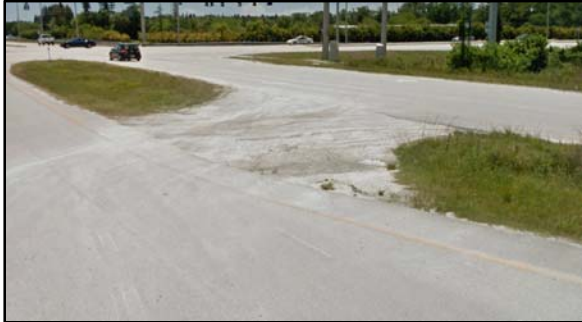
Picture 10: Evidence of Vehicles Making Southbound Left-Turns from Gas Station on Boynton Beach Blvd
