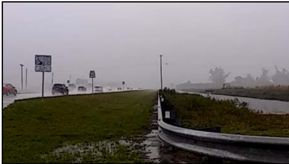
Picture 2: Guardrail and Ditch on East Side of SR-7/US-441
