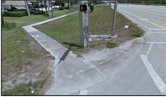
Picture 9: Curb Ramp at the Intersection of SR-7 at SR-804
