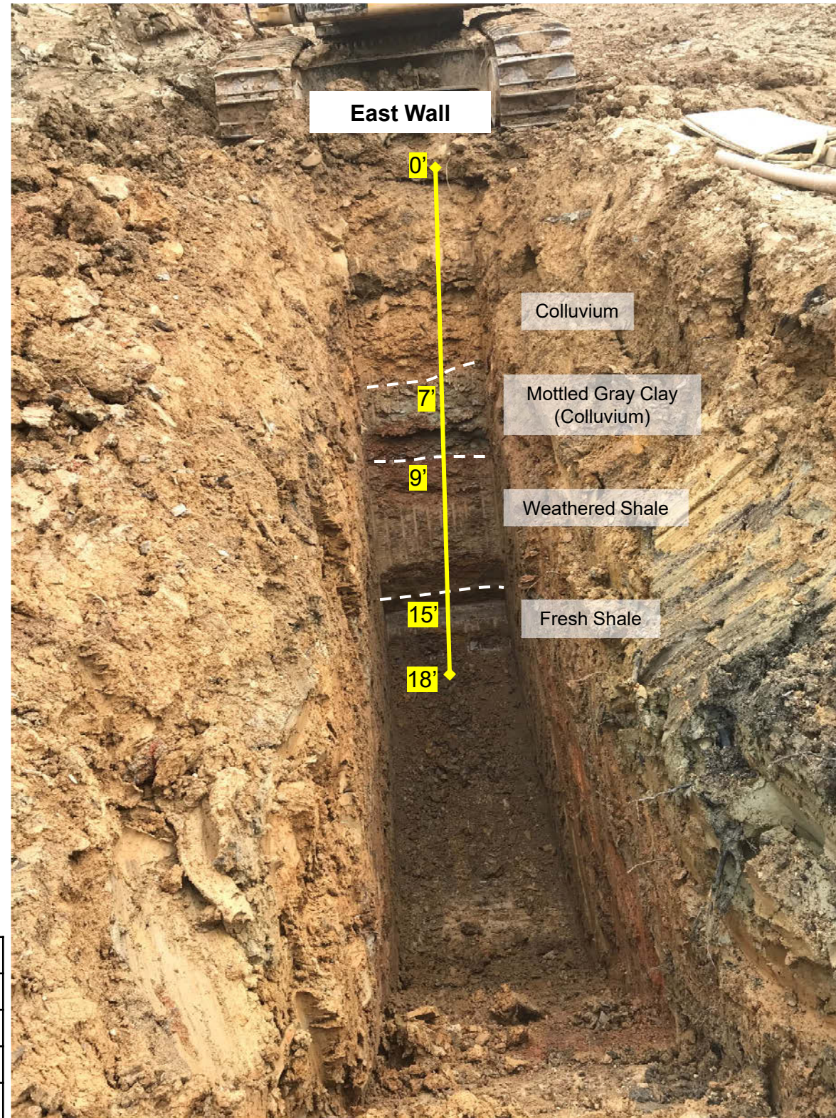
Test Pit 6A: Photo log showing fresh shale exposed at the base of the excavation.
