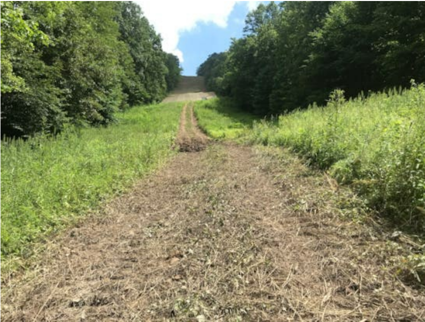
Standing near Line 25 strain 23, looking upslope at main slope.
