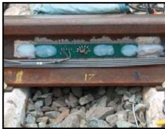
Figure 2: A Typical Strain Gage Installation on Rail Web over a Crib
