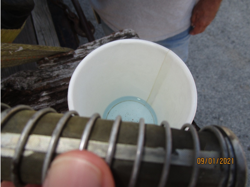
Main fuel strainer, was clear with very little debris noted
