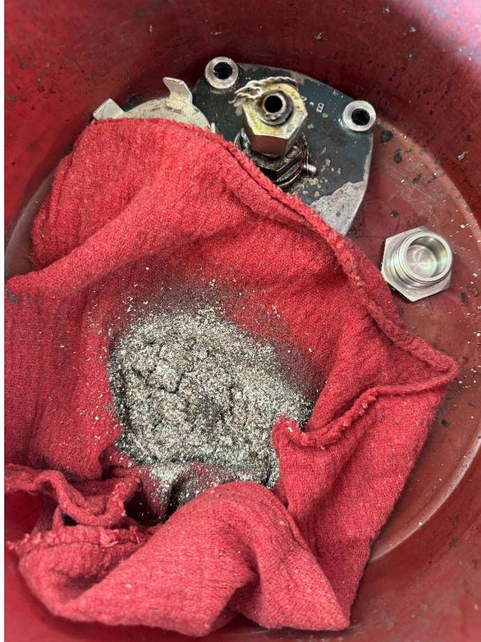
Figure 5: Main oil screen metallic debris.
