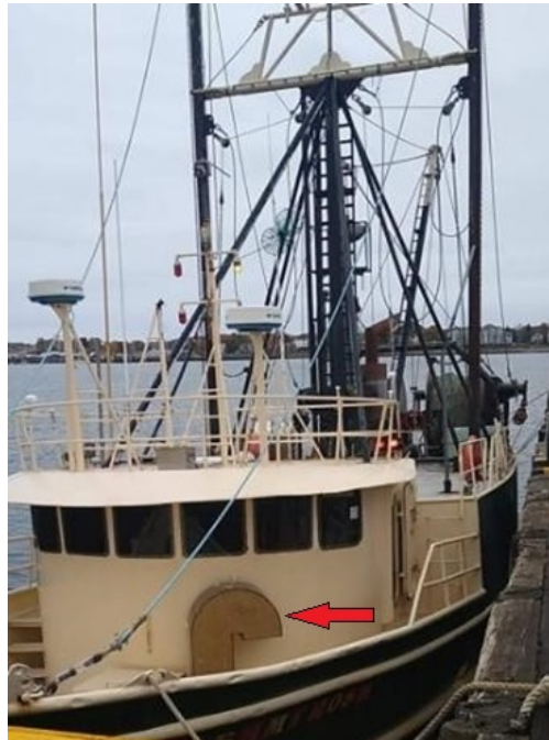
Figure 4.1: Engine Room Vent downflooding point
