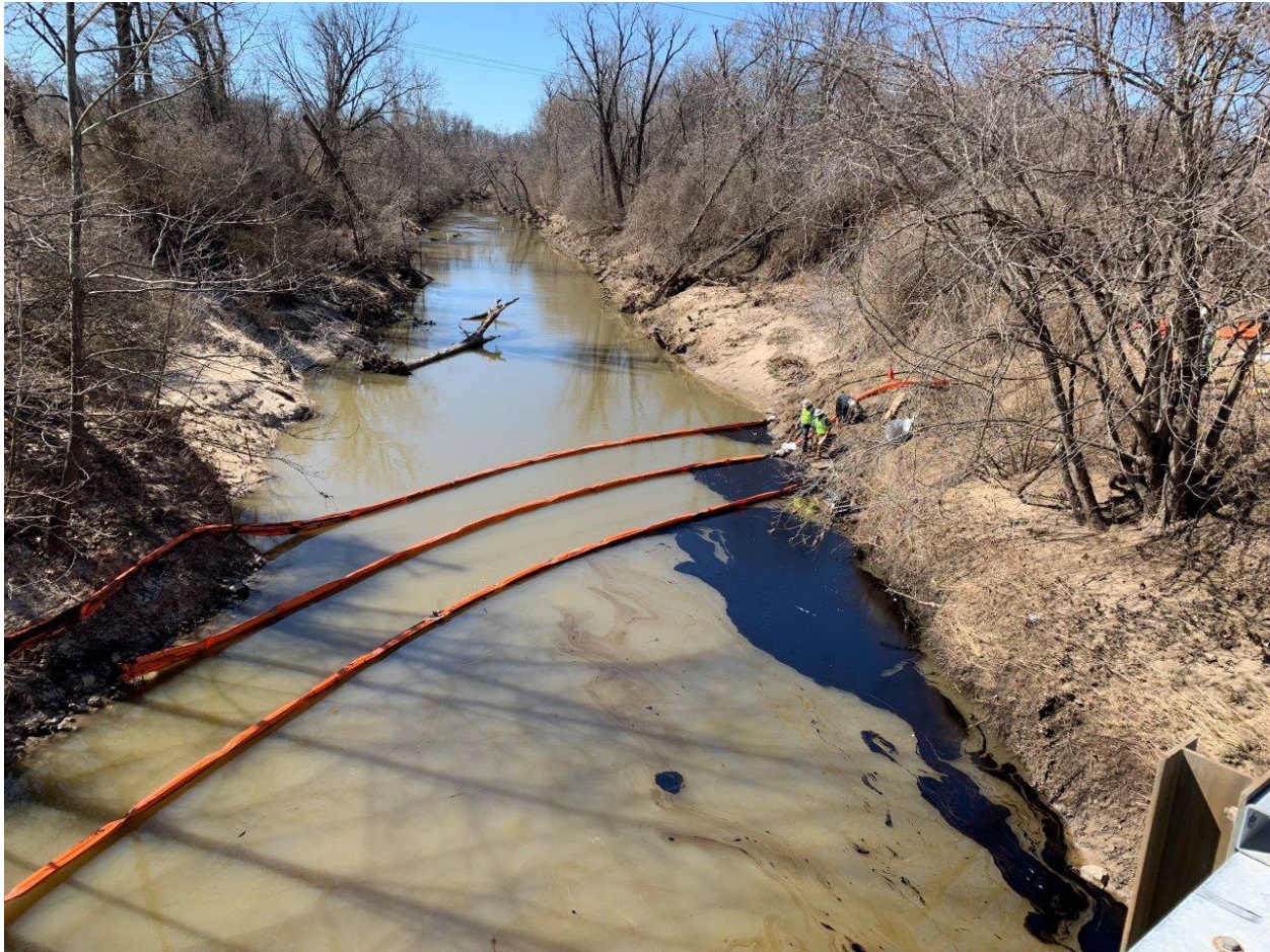
Figure. Containment booms on Cahokia Creek.
