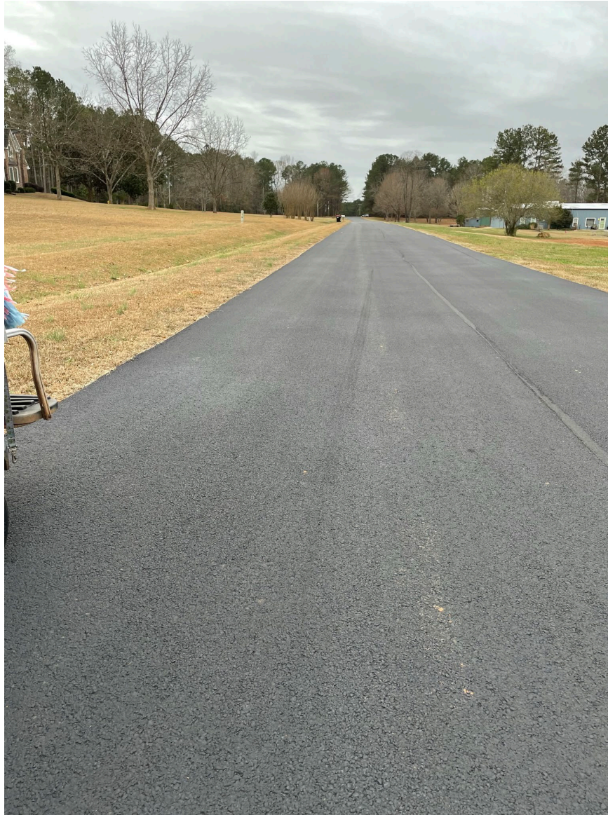
Photograph 4 - Taxiway Overview (Courtesy of FAA)
