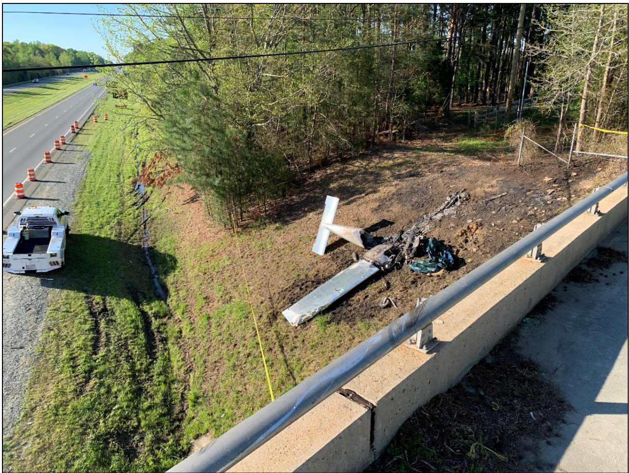
Figure 14: Overview of the accident site as viewed from the bridge the airplane impacted. Note the powerlines above the bridge, which spanned across the entire highway from east to west.
