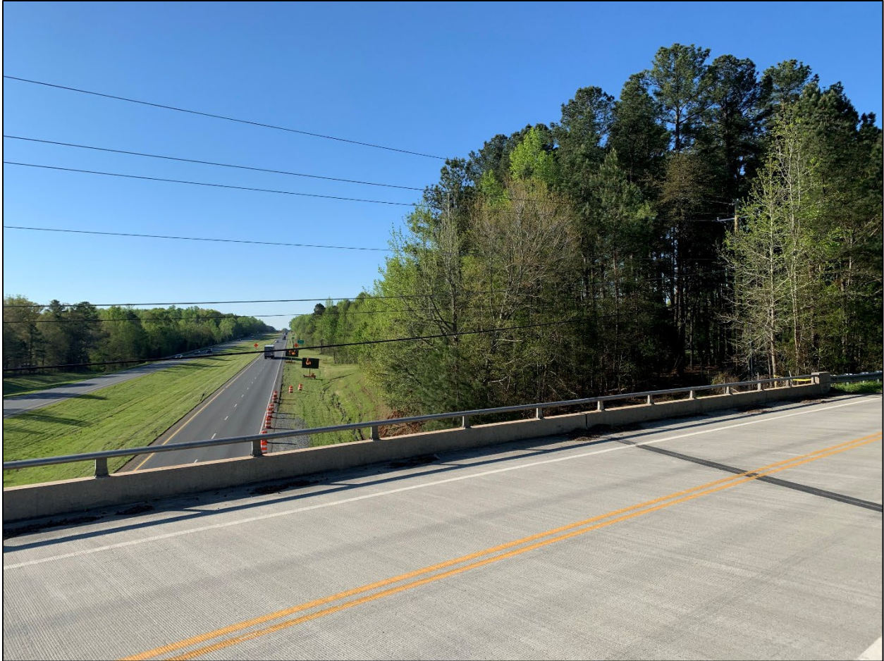
Figure 25: View of the bridge impacted and the powerlines that spanned across the entire length of the bridge across the highway. The camera is facing the direction of airplane travel and the accident site is forward and below the bridge, as referenced for this photograph.
