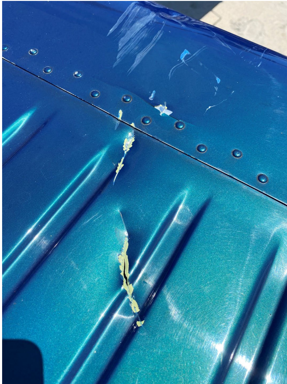
Photo 6 – Close-up view of horizontal stabilizer damage (Phot Courtesy of FAA)
