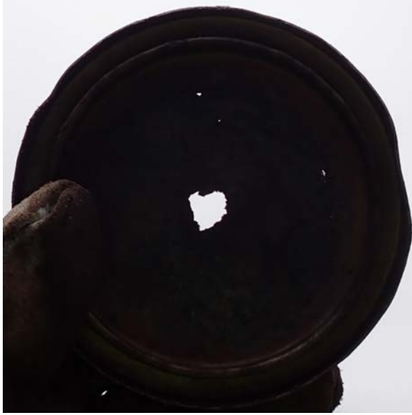
Photo 6: Muffler end plate showing corrosion
