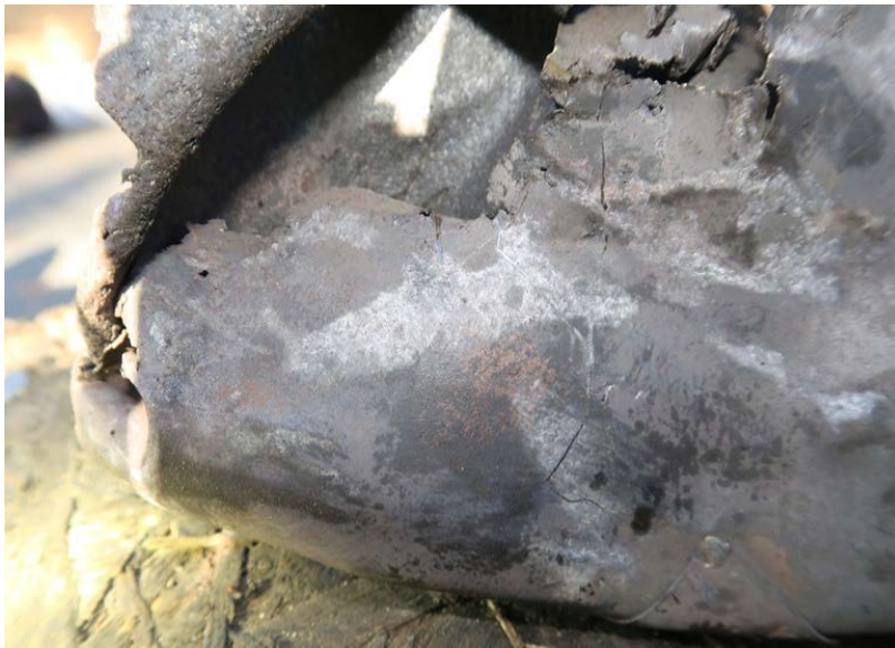
Photo 5: Muffler corrosion after muffler shroud removed
