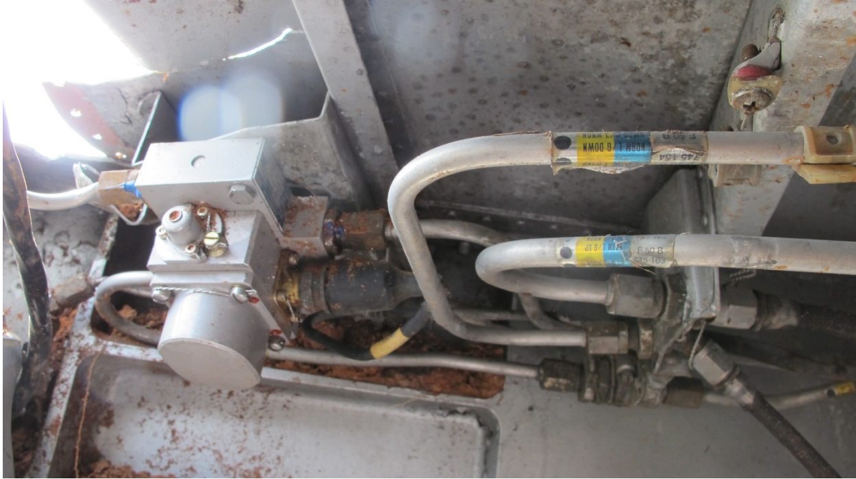
Figure 22 - LH Servo valve installed
