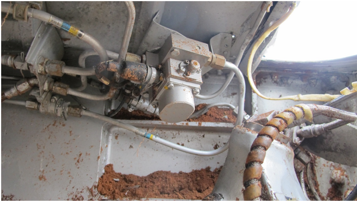
Figure 21 - RH Servo-Valve as installed
