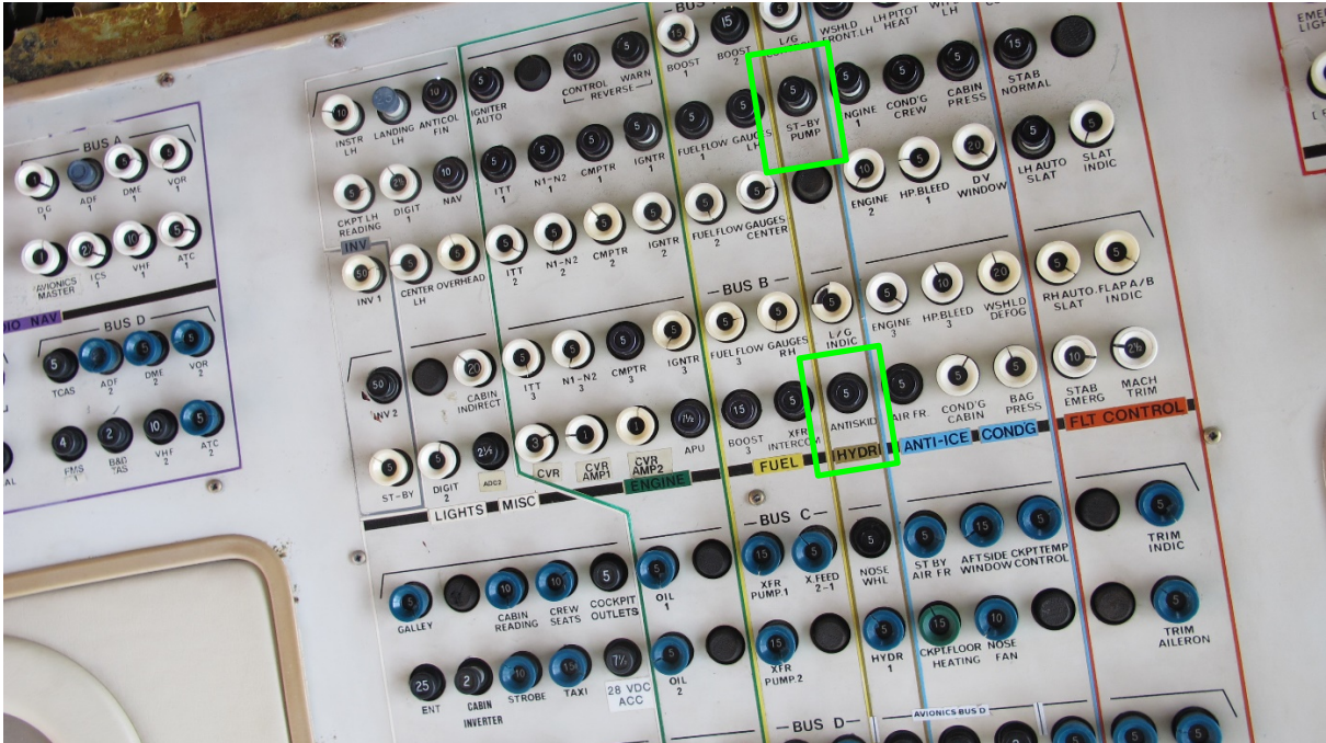
Figure 8 – Overhead C/B Panel with antiskid and standby pump breaker highlighted
