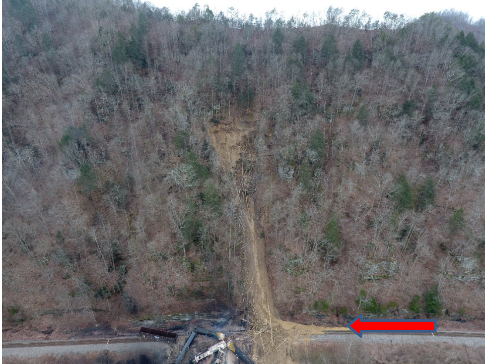
Figure 2. Aerial photo of the point of collision site taken on February 14 th . View looking at scar created by the extensive mud slide—arrow shows train direction (source: CSX drone still image)
