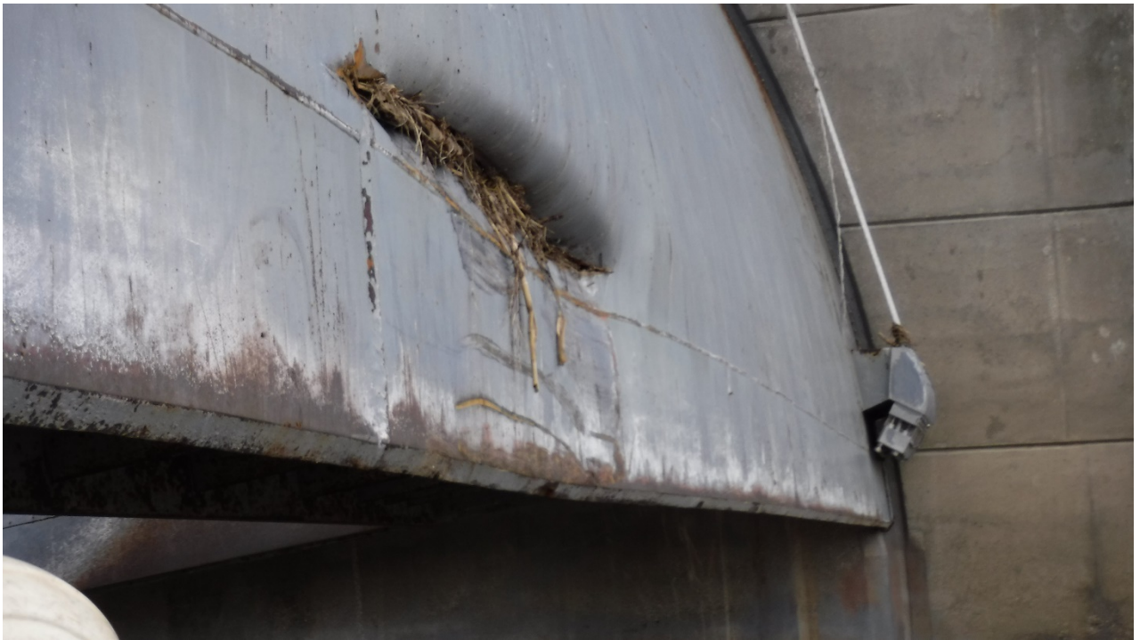
Photo 3- Tainter Gate #5 – Perforated Skin Plate
