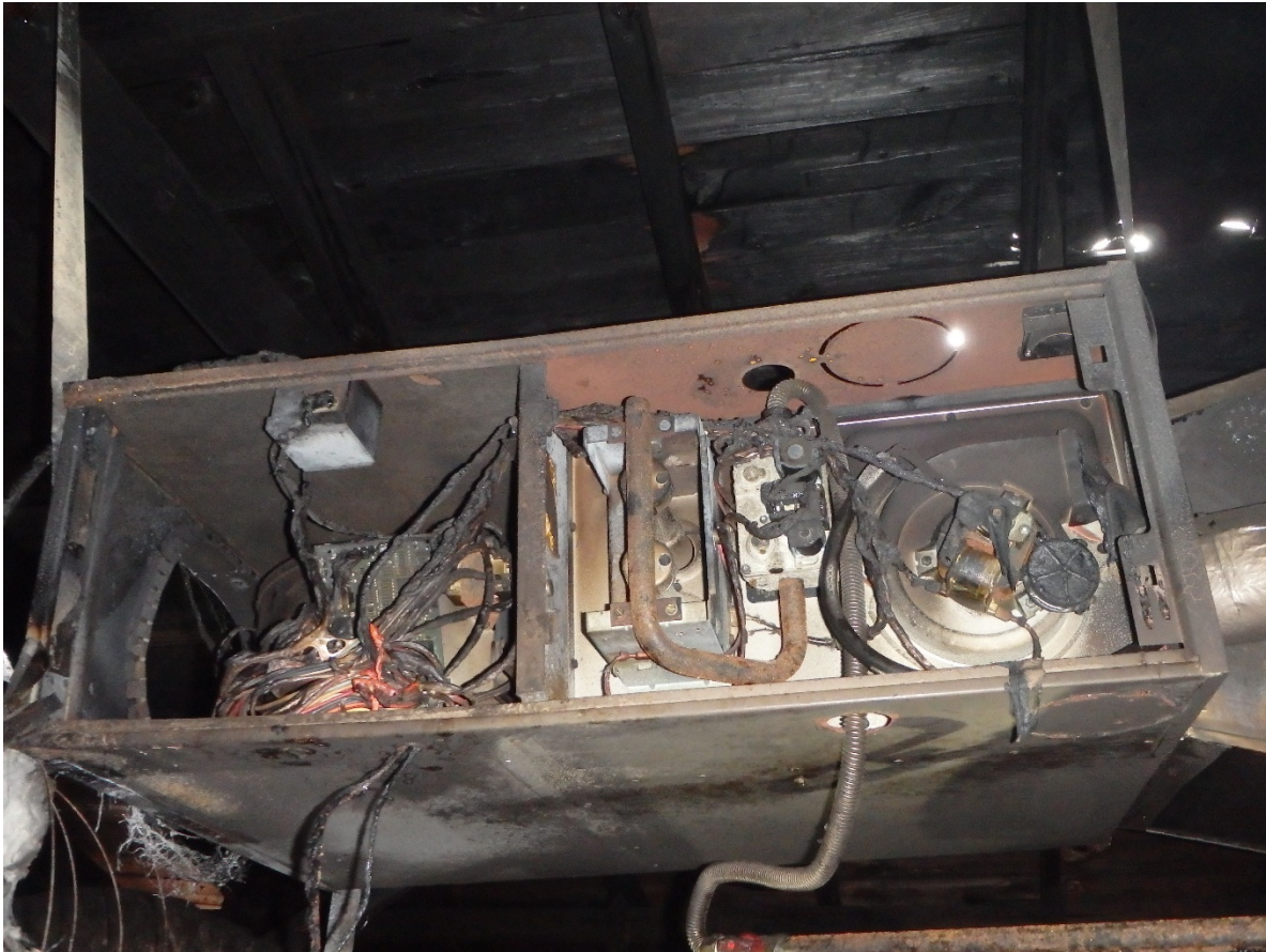
Figure 4: Post-incident photo of the furnace in 3527 Durango Drive on February 21, 2018. (Courtesy of DFR)
