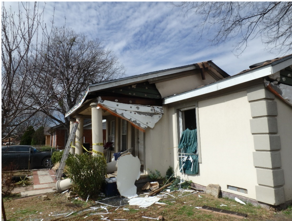
Figure 5: House 3527 Durango Drive after the February 21, 2018 incident 23
