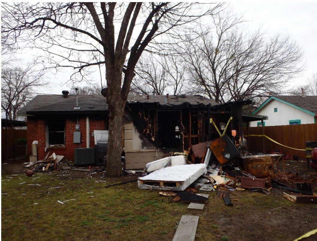
Figure 6: The back of house 3515 Durango Drive after the fire on February 22, 2018. 30
