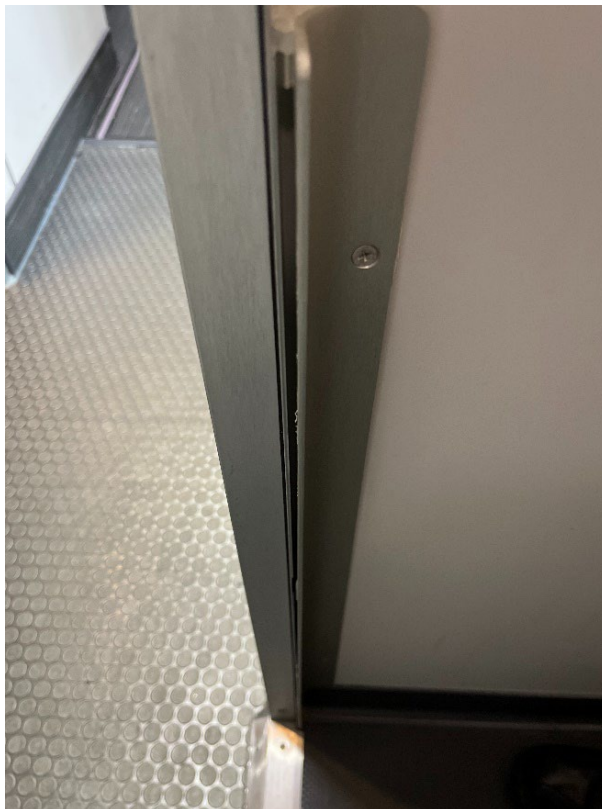
Figure 39. Trim separation from the Lav A door frame.
