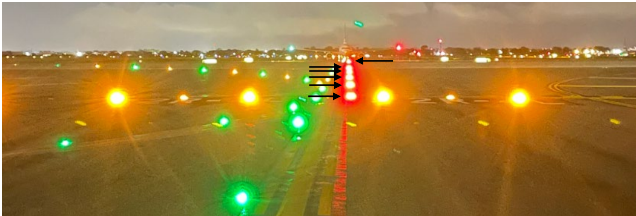
Figure 13. Photograph of activated REL lights from taxiway J crossing runway 22R-4L at night. [Source: Port Authority of NY & NJ]
