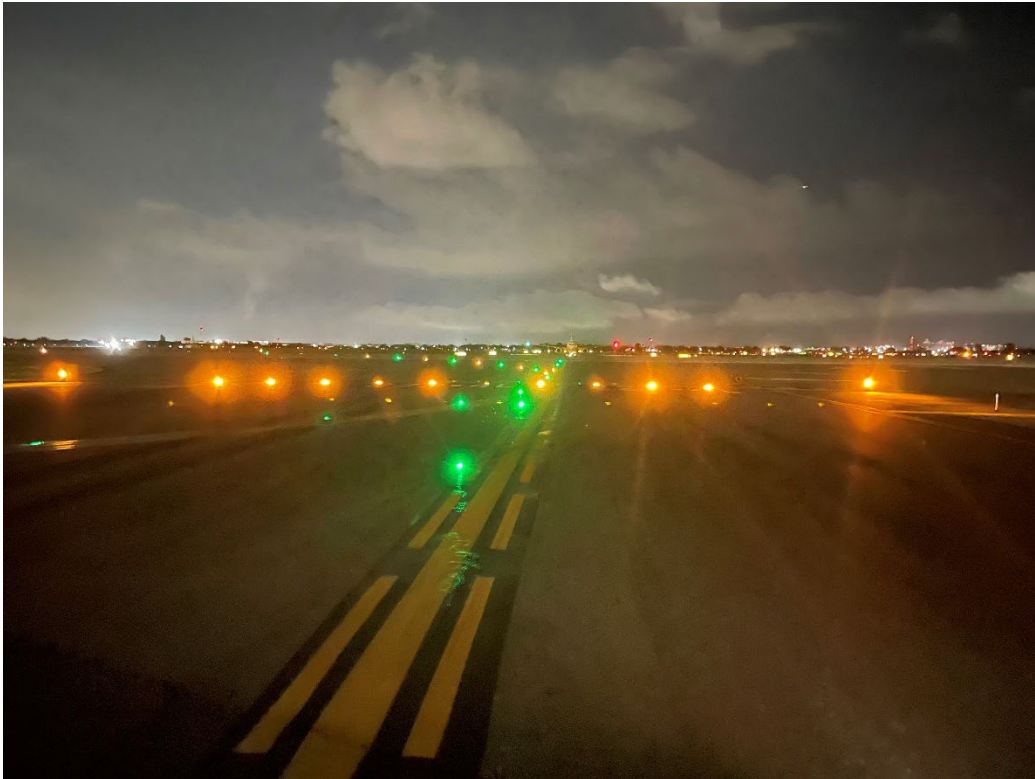
Figure 14. Nighttime photo taken just prior to the hold short marking at the taxiway J/runway 4L intersection. The taxiway centerline lights are green while the runway guard lights appear yellow/orange. [Source: Port Authority of NY and NJ.]
