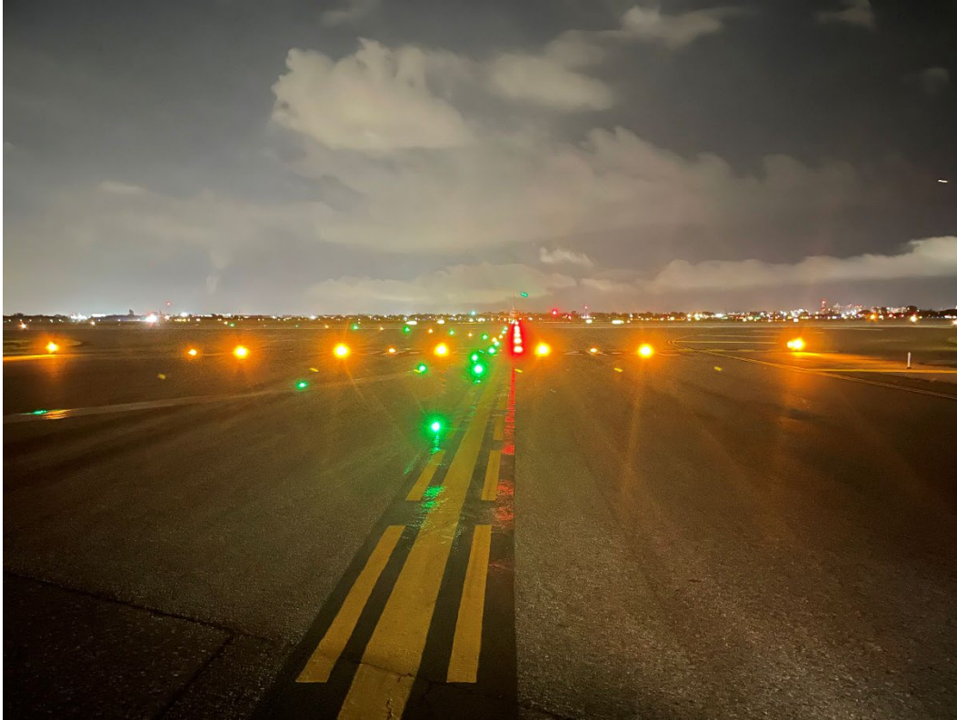
Figure 15. Nighttime photo just prior to the hold short marking at the taxiway J/runway 4L intersection with the runway entrance lights illuminated in red. [Source: Port Authority of NY and NJ.]
