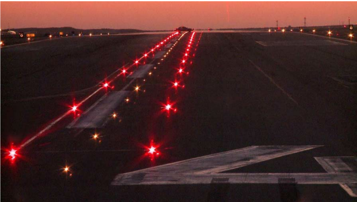
Figure 10. Illuminated red takeoff hold lights at dusk. [Source: FAA]
