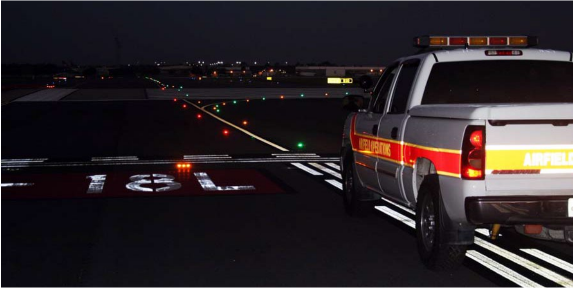
Figure 9. Illuminated red runway entrance lights at night. [Source: FAA]
