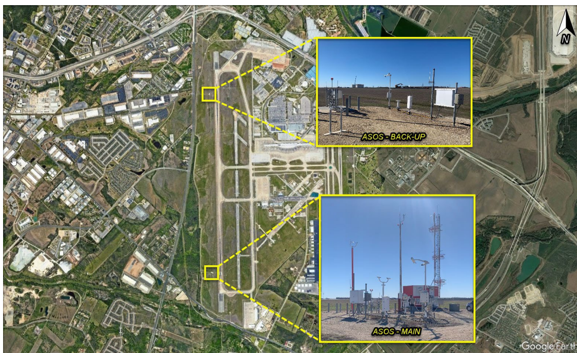
Figure 2 - Location of the main ASOS equipment and backup sensor arrays at KAUS.
