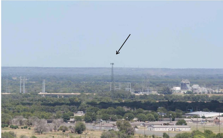
#21 1½ NE – Cell Tower (Day/Night)
