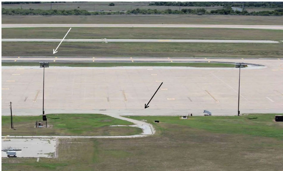
#4 1/4W – Nearest Edge of Maintenance Ramp (Day) / Lights (Night)
