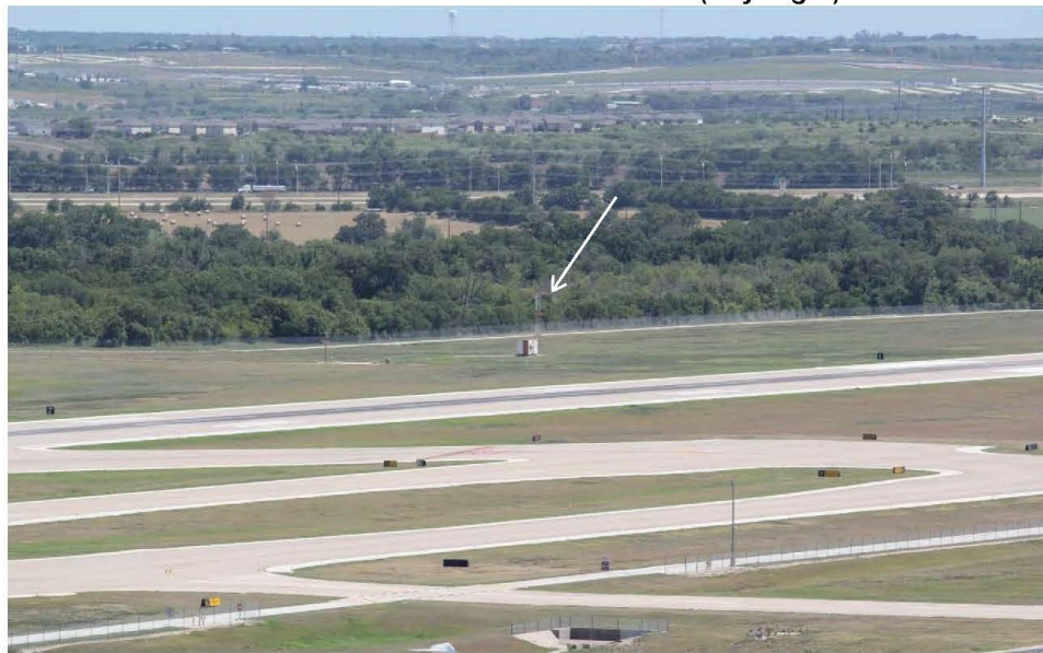
#12 1 SE – RWY 36R Glideslope Building (Day/Night)
