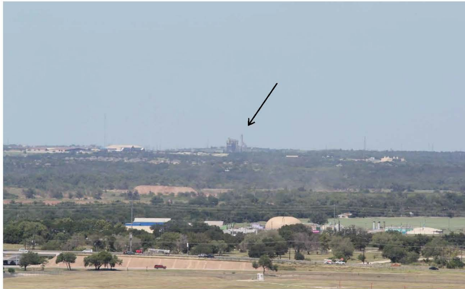
#17 8 N – Decker Creek Power Plant (Day/Night)
