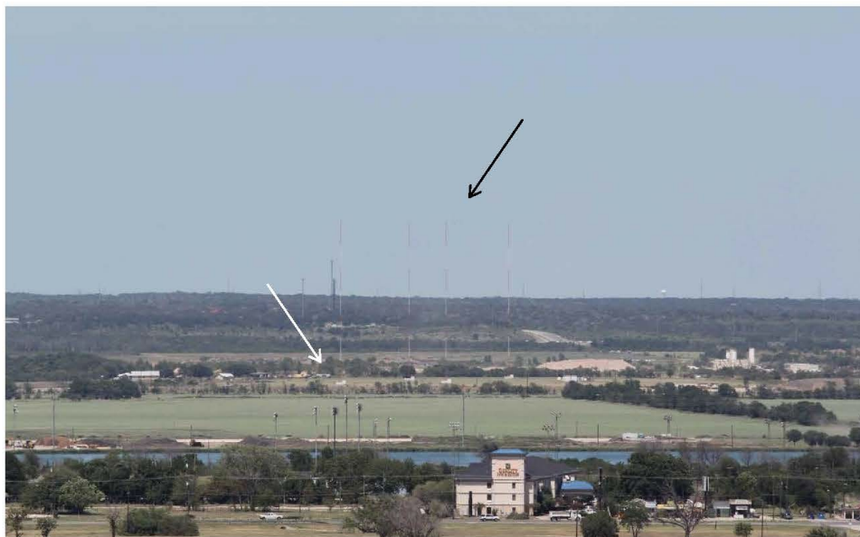
#5 3 NE – KLBJ Antenna Buildings (Day) / Lights (Night)
