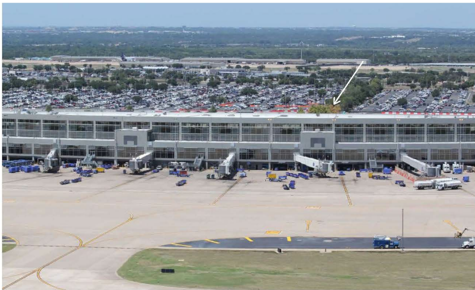
#6 1/2 N – Nearest Side of Terminal Building, NOT Gates (Day/Night)
