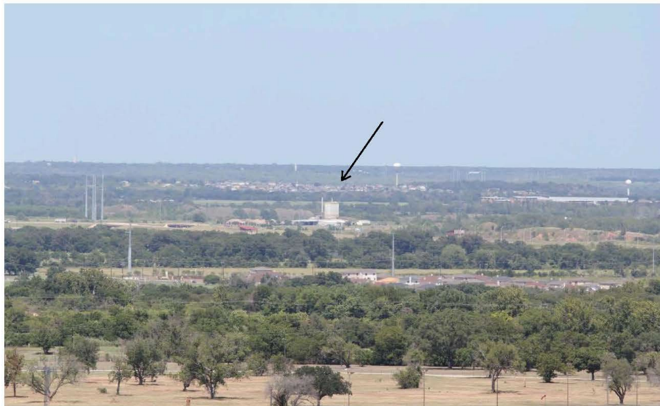
#9 4 NE – Block Building of Texas Industries (Day/Night)
