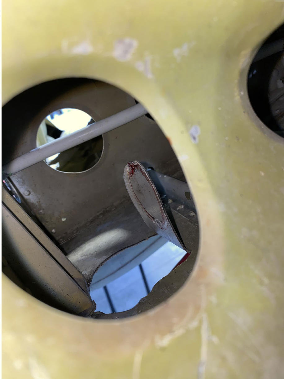
Figure 7. Lower stabilizer skin punch through and grease imprint (NTSB photo)
