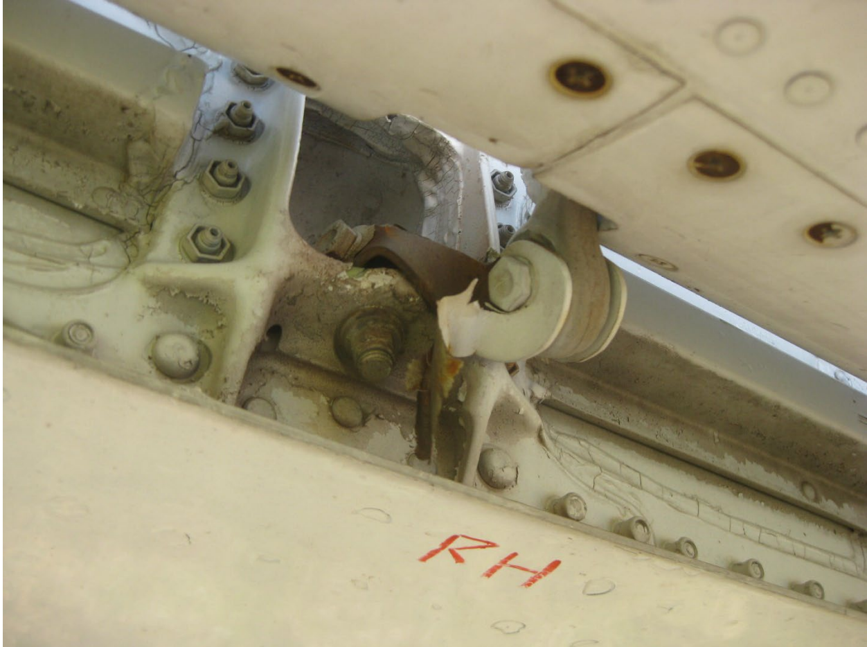
Figure 28. Right elevator inboard geared tab attachment linkage, looking forward (into the horizontal stabilizer) and outboard, viewed from underneath the right elevator.
