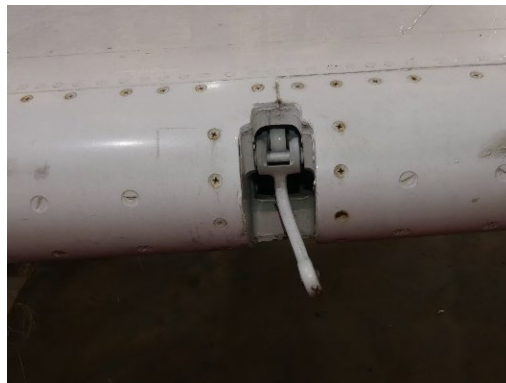
Figure 43. The left geared tab inboard input crank (looking aft). Note that the crank is bent outboard.
