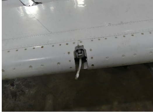
Figure 44. The right geared tab inboard input crank (looking aft). Note that the crank is bent outboard.
