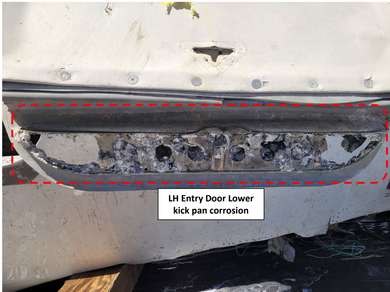
Figure 35. Left Forward Entry Door lower kick pan corrosion (Boeing photo)
