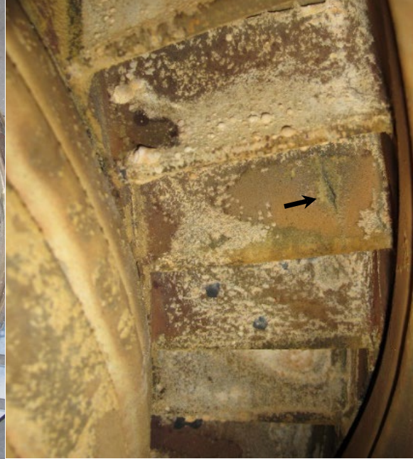
Figure 36 Chordwise vane crack
