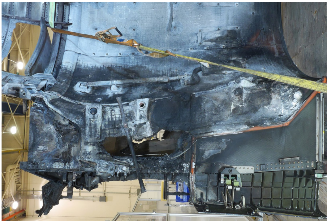
Figure 16 - Inboard thrust reverser lower bifurcation with blankets installed
